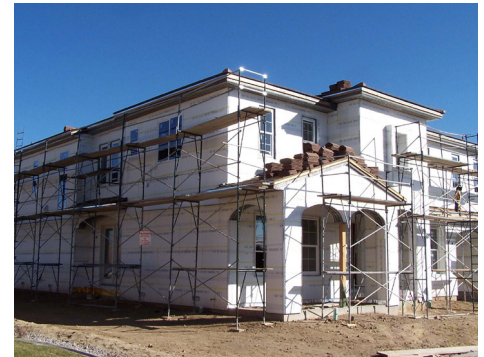
CONTINUOUS EXTERIOR INSULATION
